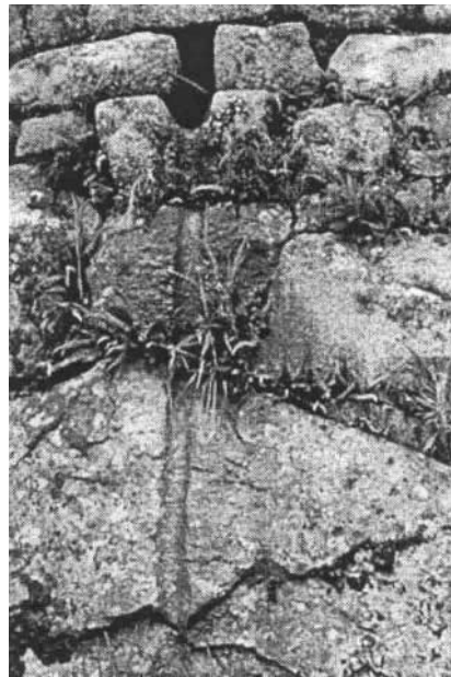
Figure 10. Engineers Strategically Placed 129 Surface Drainage Outlets in Walls to Drain Interior Ground Surfaces. This Drainage Outlet Was Fitted with Vertical Channel to Avoid Splash.
